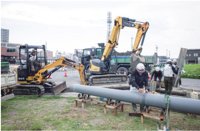
Water pipe installation
