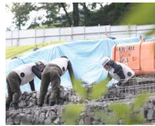
Civil engineering work
